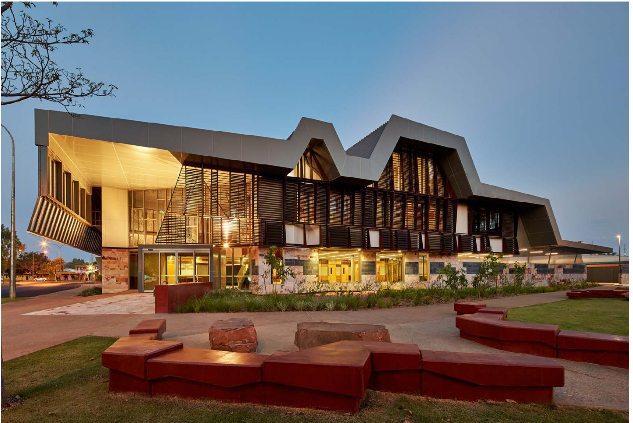
Kununurra Courthouse. With TAG Architects
